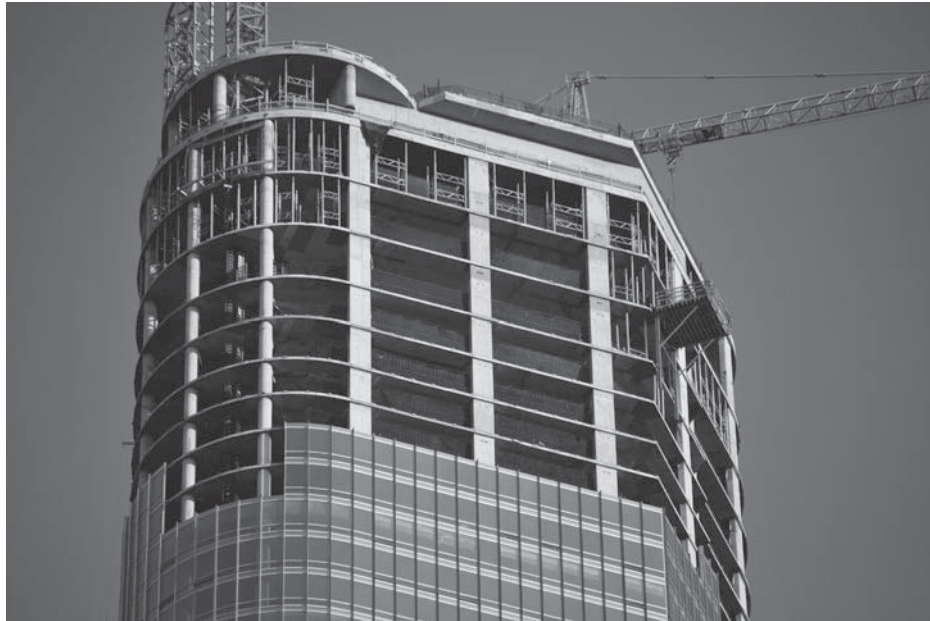
Fig. 1-1 Trump Tower of Chicago. (Photograph courtesy of Larry Novak, Portland Cement Association.)
